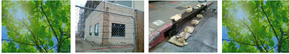
New School Construction site near 70th Street and Vermont Avenue
